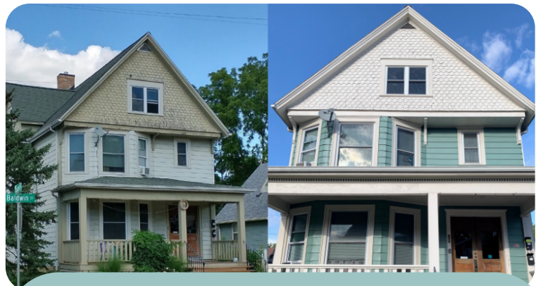
A before and after shot of our 601 S Baldwin St. property. Refinishing the exterior was only financially feasible because of the Capital Improvement for Non-Profit Housing Grant.
